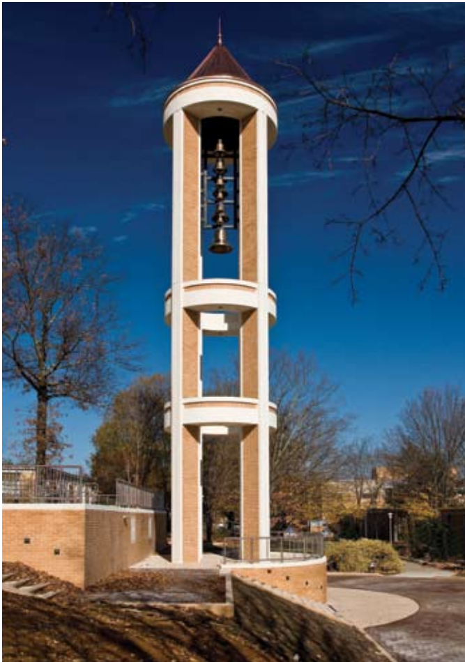
Fig. 3: The architectural precast elements for the bell tower at Dalton State College were produced by Metromont Corporation
